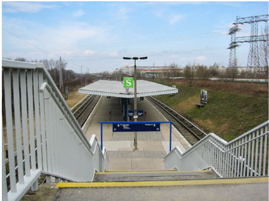
Foto: DB Station&Service
